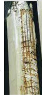
*Deterioration of concrete due to improperly designed rebar splices and lack of reinforcement, often leads to premature splice failure.*
