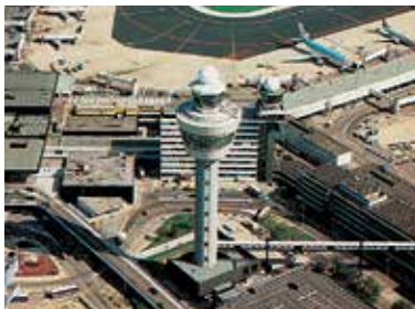
Control tower, Schiphol Airport – Amsterdam
