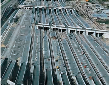
Channel Tunnel Terminal, UK
