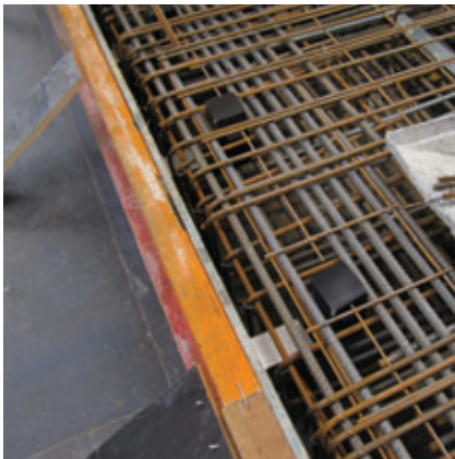
Reinforcement being located around ESDQ-L20 Sleeves
