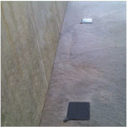
Void formers shown at Slab-to-Wall joint
