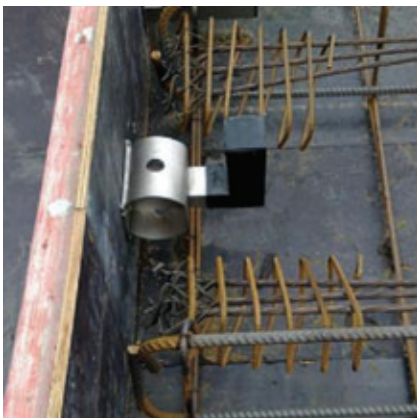
HLDQ-L30 Sleeve nailed to formwork
