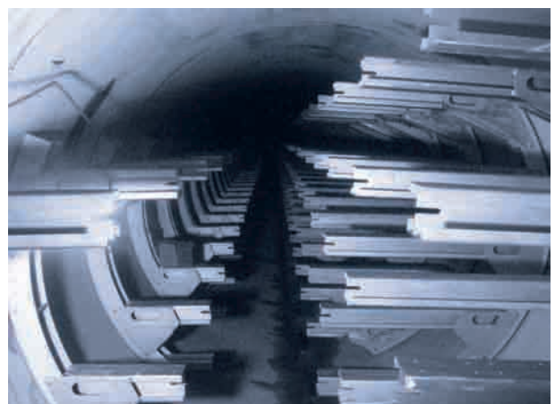
Project: Carlton Cable Tunnel, Australia (Client: Energy Australia, Contractor: The Abergeldie Group, Cable Support Engineering: Ancon)
