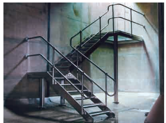
Access Walkways and Ladders
