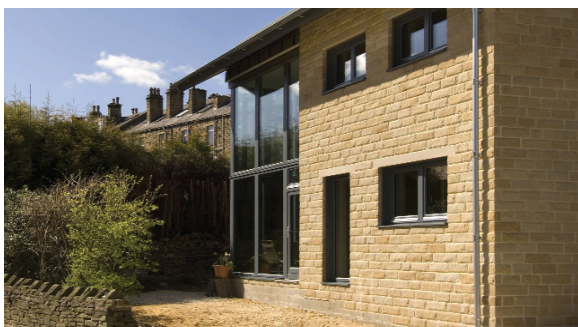
© Green Building Store
