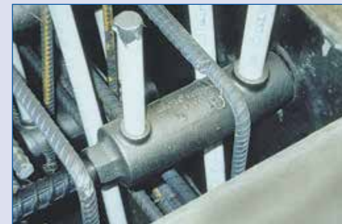
Standard 1/2" (13 mm) and 3/4" (19 mm) PVC or flexible tubing is used for the inlet and outlet ports.
