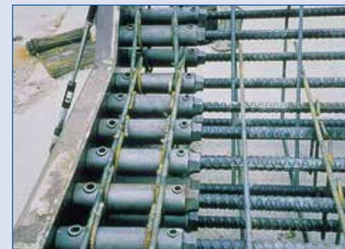
The taper threaded sleeve keeps the bar in axial alignment to increase field tolerance of the rebar dowels.
